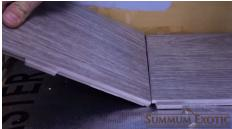
2- The last plank of the other rows must be installed with a hammer with a 45° angle. The plank can than be slipped in using a hammer and a pull bar.
