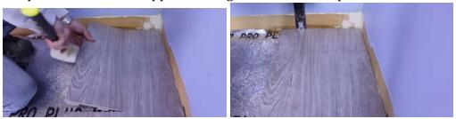
3- At the end of every row, insert spacers between the plank and the wall to stabilized your row.
